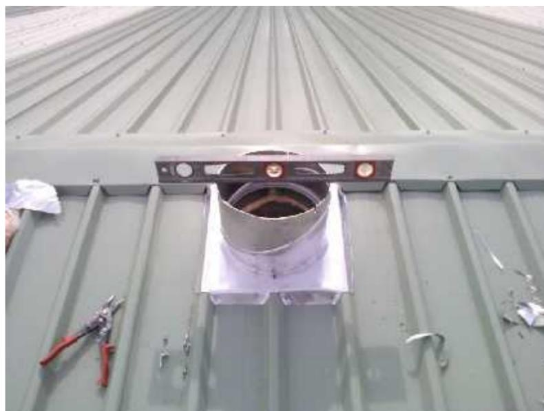
Use a spirit level and 4 point level the unit, this is important to ensure operation into the wind
