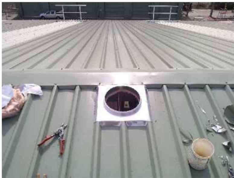
Shape flashing base to roof profile and secure base, under ridge capping and seal with silicone.
