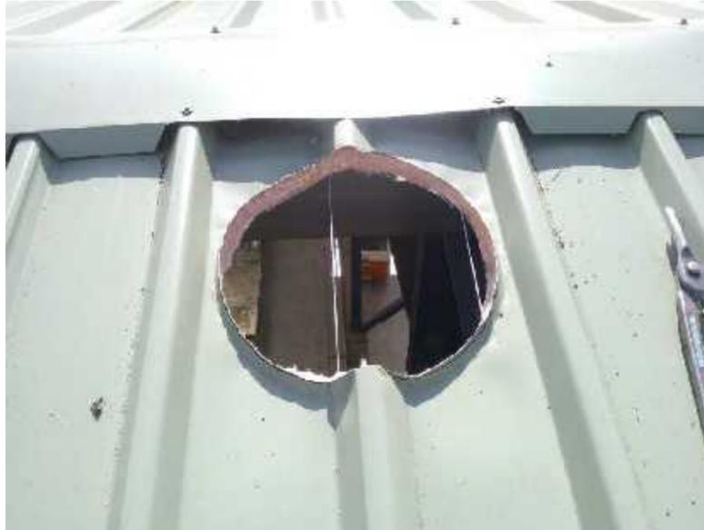
Using the base as a template cut the hole 15 mm shorter to turn up profile to form **a lip to provide a barrier for any driven rain that may penetrate under the ridge cap**, which should also have a silicone seal between it and flashing base
