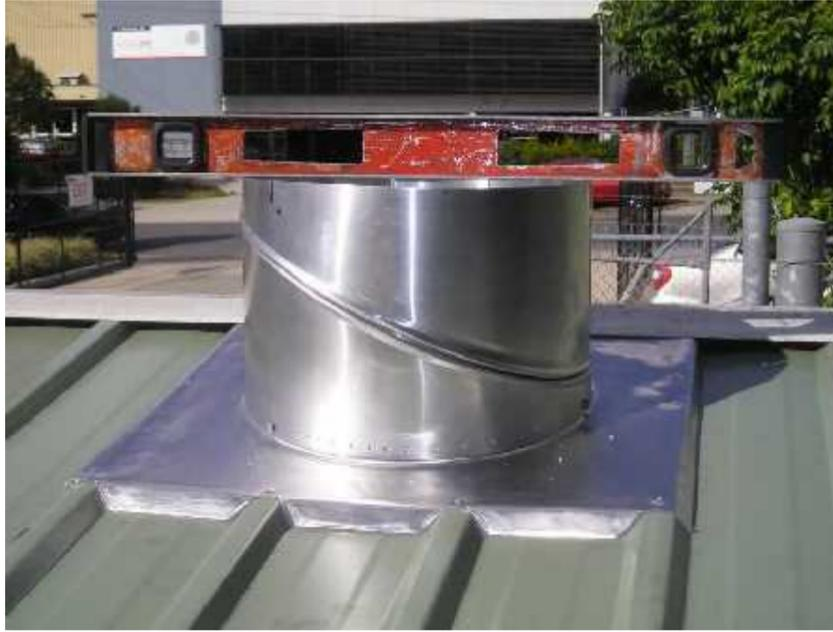
Secure flashing base with pop rivets or hex head screws with neoprene washers (not provided) and secure the varipitch to flashing base with the three neoprene clima seal washers provided at equal 1/3 spacing around the flashing base
