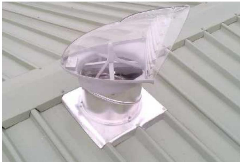
Secure head of unit by lining up pre drilled brackets and fix with hex screws (without neoprene washer) provided
